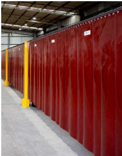
Figure 10: Strip type welding bay curtains. The curtains will not be able to slide along the rail at the top. It will be possible to remove individual strips for replacement.
